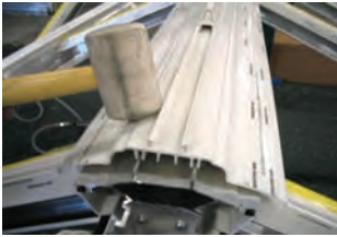
Centralise the two clips on the ridge top cap with the two barbs on the main ridge.
