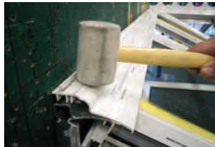
The PVC-U wallplate top cap is exactly half of a ridge top cap and is fastened in the same manner.
